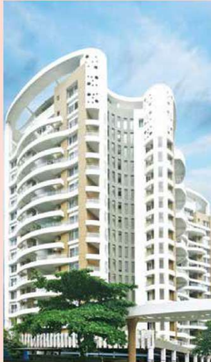
Plaadium, Pune by Encraft
